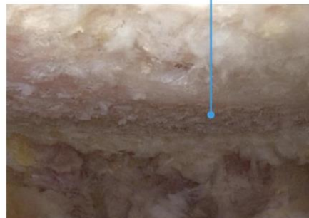
After Milling / Smoothing the Bony Shoulder Roof
